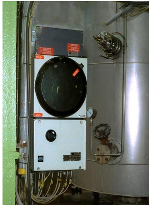
NDU electronics in ex - proof housing
